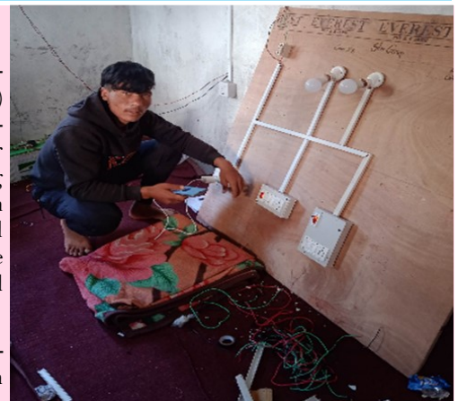
One of the trainees practicing in house wiring training.
