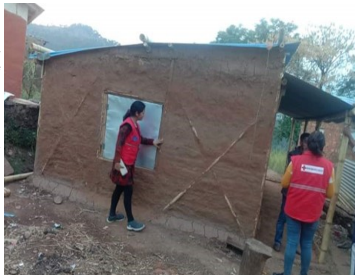
Newly constructed transitional shelter through CVA modality in Mangalsen Municipality, Achham district
