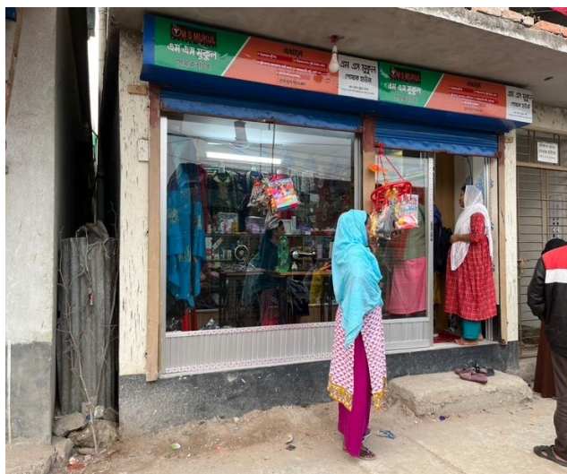
Caption: Examples of measures taken to protect a shop premises and home (both of programme participants) by raising the plinth above ground level.
