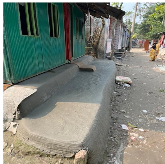
Caption: Examples of measures taken to protect a shop premises and home (both of programme participants) by raising the plinth above ground level.
