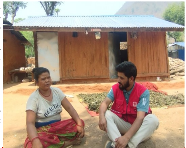
Newly constructed transitional shelter through CVA modality in Bheri Municipality, Jajarkot district
